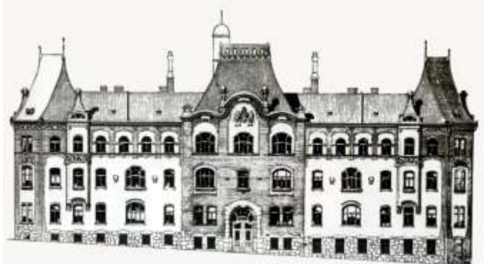
The Headquarters of the Hungarian Meteorological Service by the original plans from 1910
